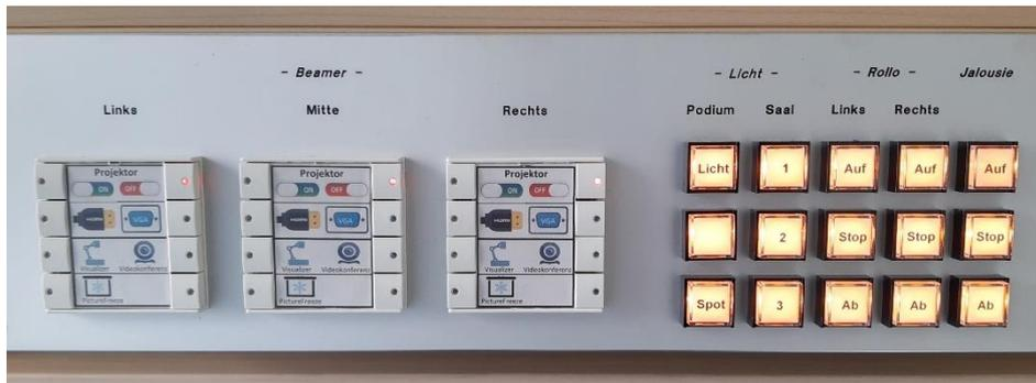
The three controls on the left represent the three installed beamers. An indicator light shows the status.
